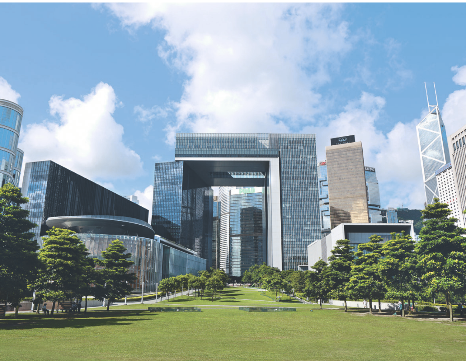
From right: The Office of the Chief Executive of the Hong Kong Special Administrative Region (HKSAR), the Central Government Offices of the HKSAR Government and the Legislative Council Complex.
